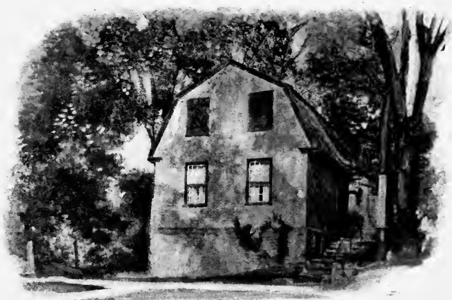
Old Brick Schoolhouse, Norwich, Connecticut
